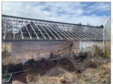
Figure 9: Greenhouse with no roof canopy and exposed metal framing.
