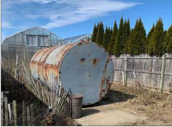
Figure 7: Above ground storage tank with visible rusting
