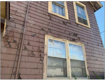
Figure 4: Existing conditions of windows with cracking to the window sills.
