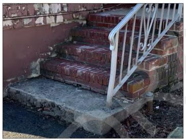
Figure 3: Deterioration of front steps.
