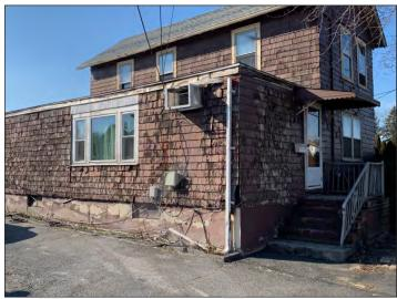
Figure 2: Side of house with evidence of cracking on foundation wall.
